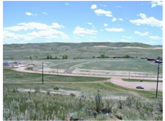
Native plants such as western wheatgrass, galleta, and blue grama were installed on the surface of the 15-acre evapotranspiration cover.
