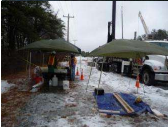
Continuous cores water table to bedrock 70 – 315 ft bgs
