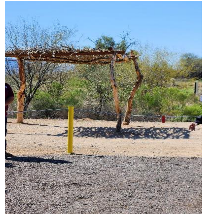
A water treatment structure. Source: Arizona DEQ
