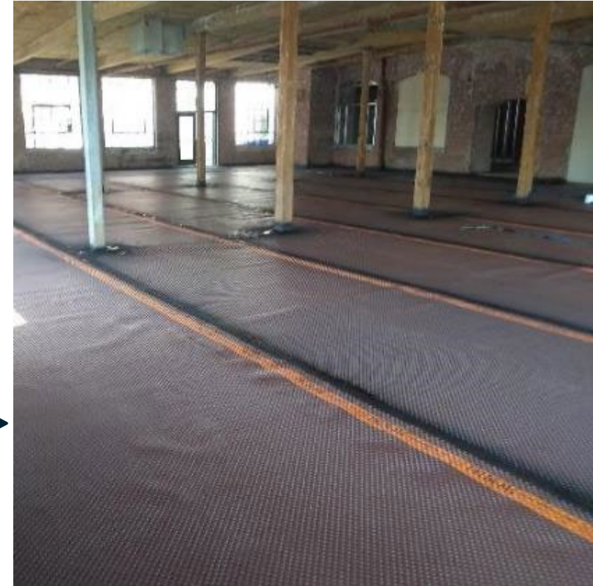
Source: Contractors Waterproofing, 2021. Used with permission.
