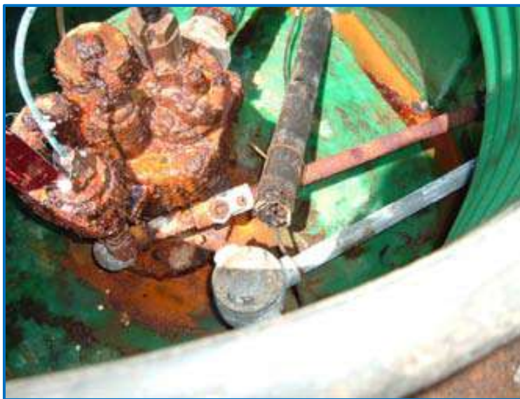
Corroded STP
