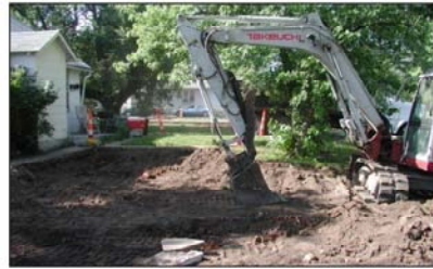
Post-Excavation Confirmatory Sampling
