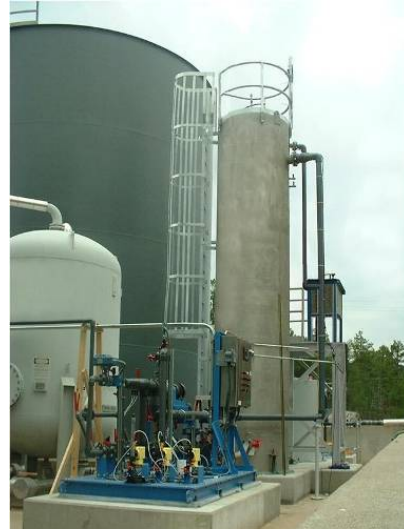
Fluidized Bed Reactors at Longhorn Army Ammunition Plant, TX
