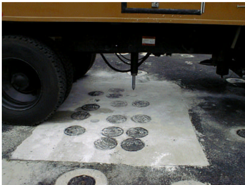
Figure 8-9. Core Sampler Extracting Vertical Core at Dover AFB
