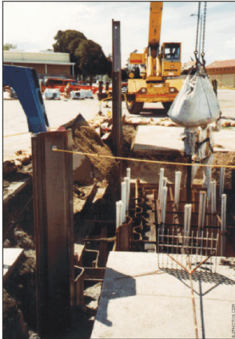
Figure 8-2. Monitoring Wells Being Installed in (a) Trench-Type and (b) Caisson-Type Reactive Cells
