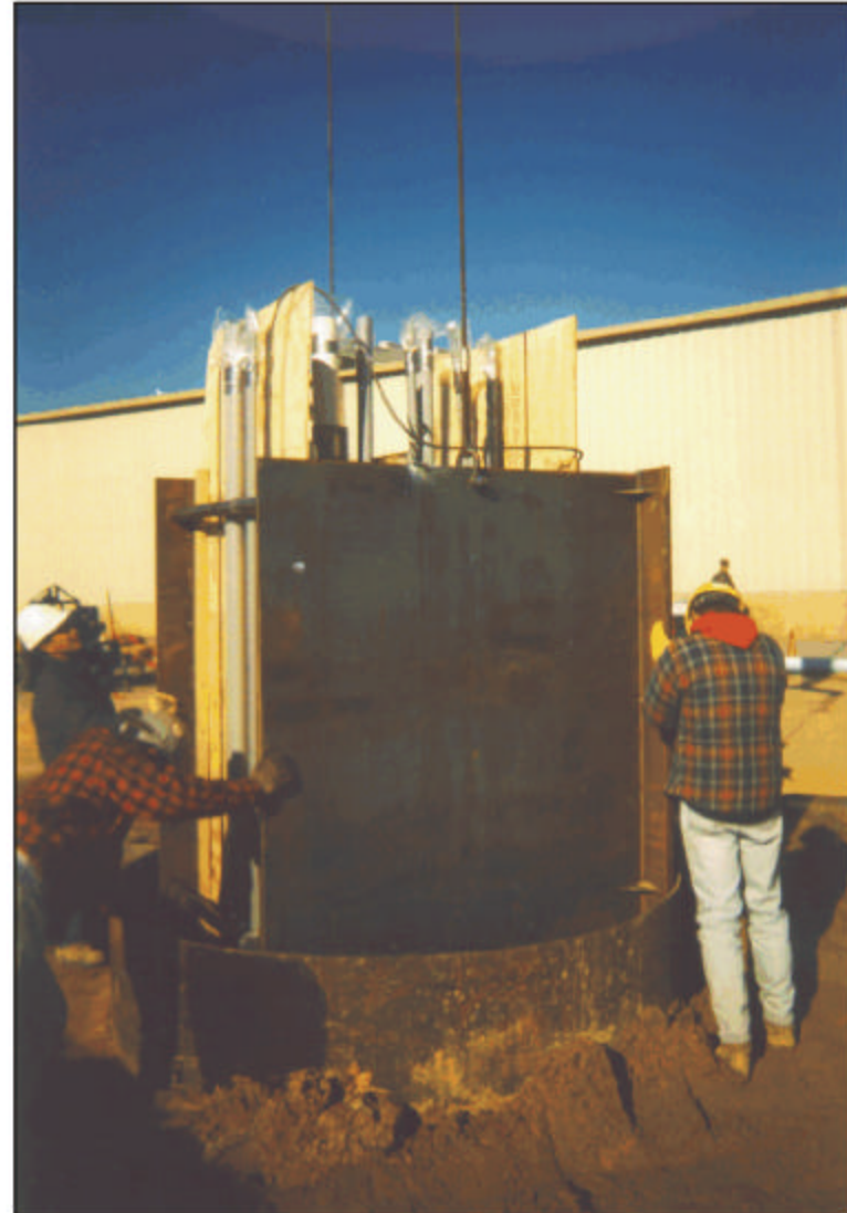
Figure 8-2. Monitoring Wells Being Installed in (a) Trench-Type and (b) Caisson-Type Reactive Cells
