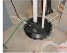
Figure J-4. Passive sump mitigation system. Photo Source: Kansas Dept. of Health and Environment
