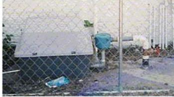
Figure 6-1. Small-scale soil vapor extraction (SVE) system designed to address the source of vapors. Photo Source: Vapor Mitigation Sciences, LLC.
