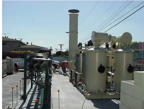
Picture from USEPA Region 9: Charnock MTBE Cleanup Project - Soil Vapor Extraction
