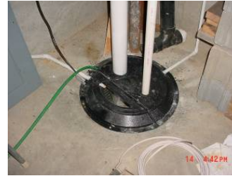
Passive sump mitigation system
