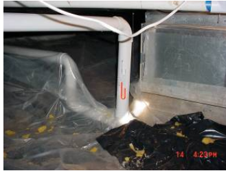
Crawlspace mitigation using sub-membrane depressurization (SMD)
