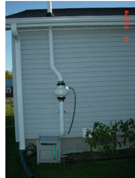
Active sub-slab depressurization (SSD) system
