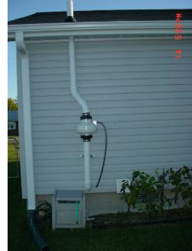
Active sub-slab depressurization (SSD) system
