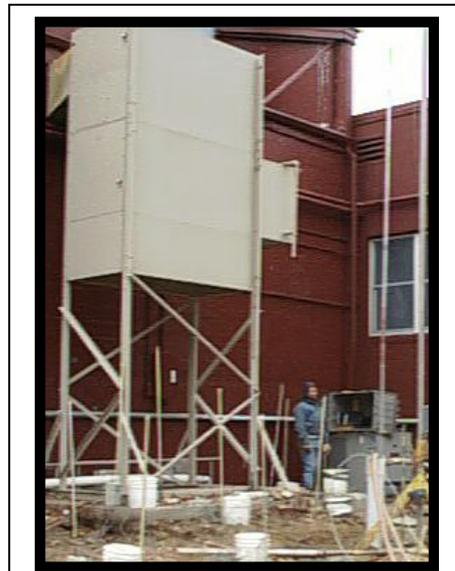
This air-handler, which was constructed on a 4-inch thick concrete pad, was elevated by fractures created at a depth of seven feet. Hydraulic fractures were created from a boring located at the lower, rightmost corner of this photograph – at the base of the yellow hoist unit. The staffs were used to measure uplift while the buckets protected tiltmeters.
