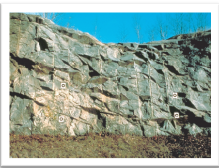
Schist : fewer fractures; longer, undulating fracture surfaces
