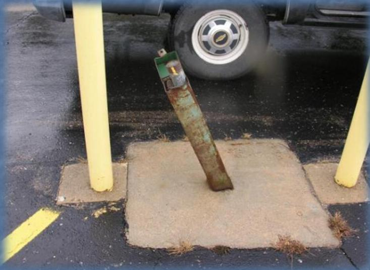
No lock or inner well cap, wasp nest, subsiding of grouting materials
