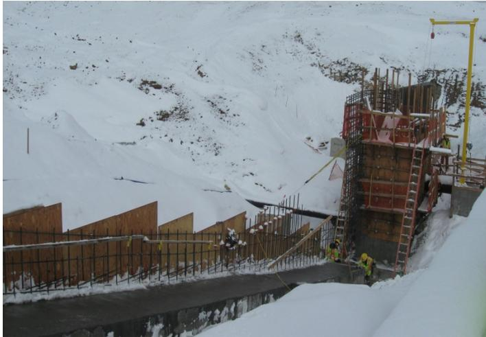
**Source Control Measures – Collection System Cut-off walls**
