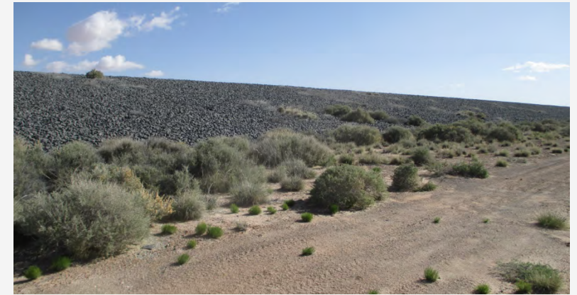
Vegetation on Tuba City UMTRA Cell Threatens Radon Barrier
