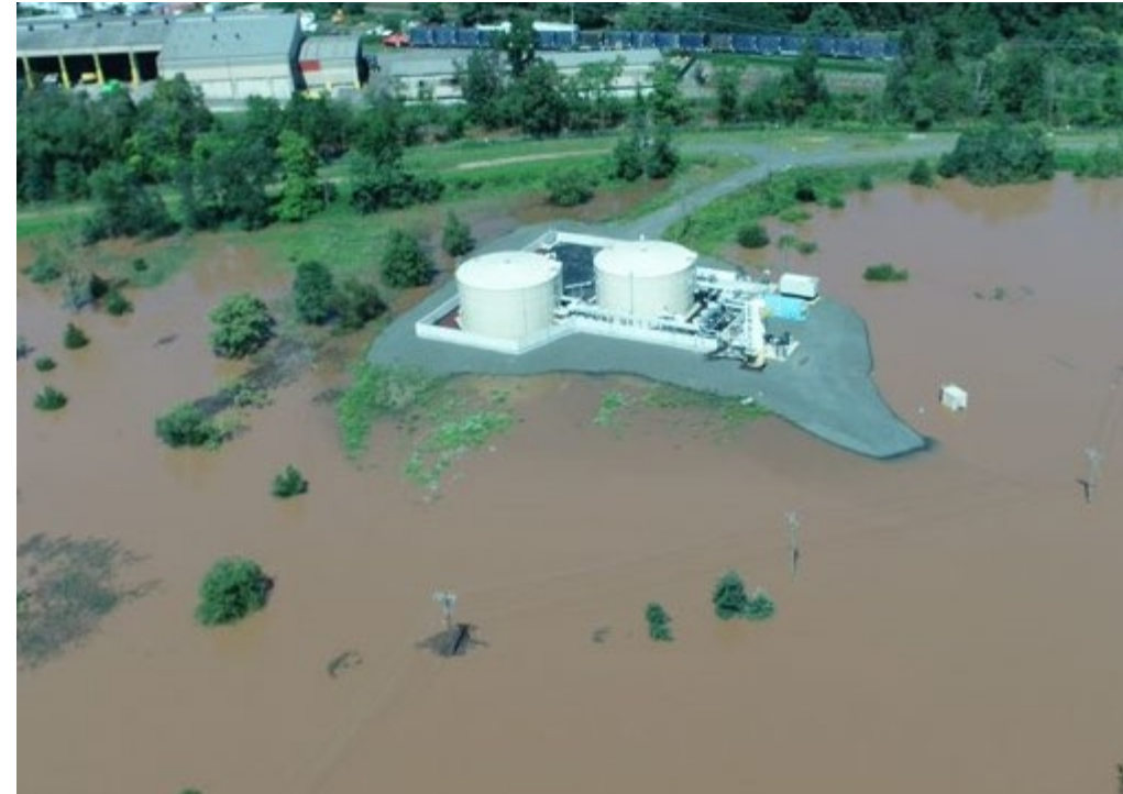
Groundwater treatment plant and storage tanks, constructed on elevated land outside of 500-year floodplain, avoided floodwaters in 2021.
