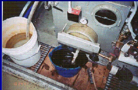
Water Treatment Unit (above) Treats separator water
