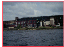
New Bedford Harbor (and other contaminated sites)
