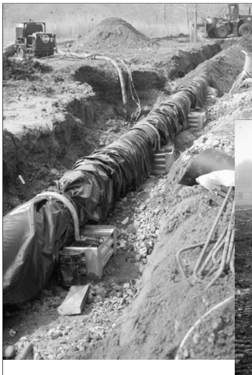
Installation of sewer pipeline across Park (City of New York)
