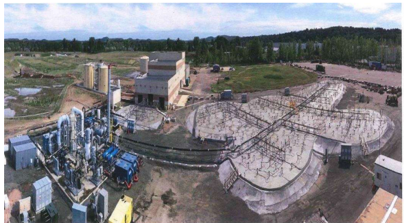
In situ thermal treatment technologies have advanced markedly, due in large part to research and demonstrations supported and conducted by FRTR Member Agencies. Photograph of the Velsicol Superfund site.
