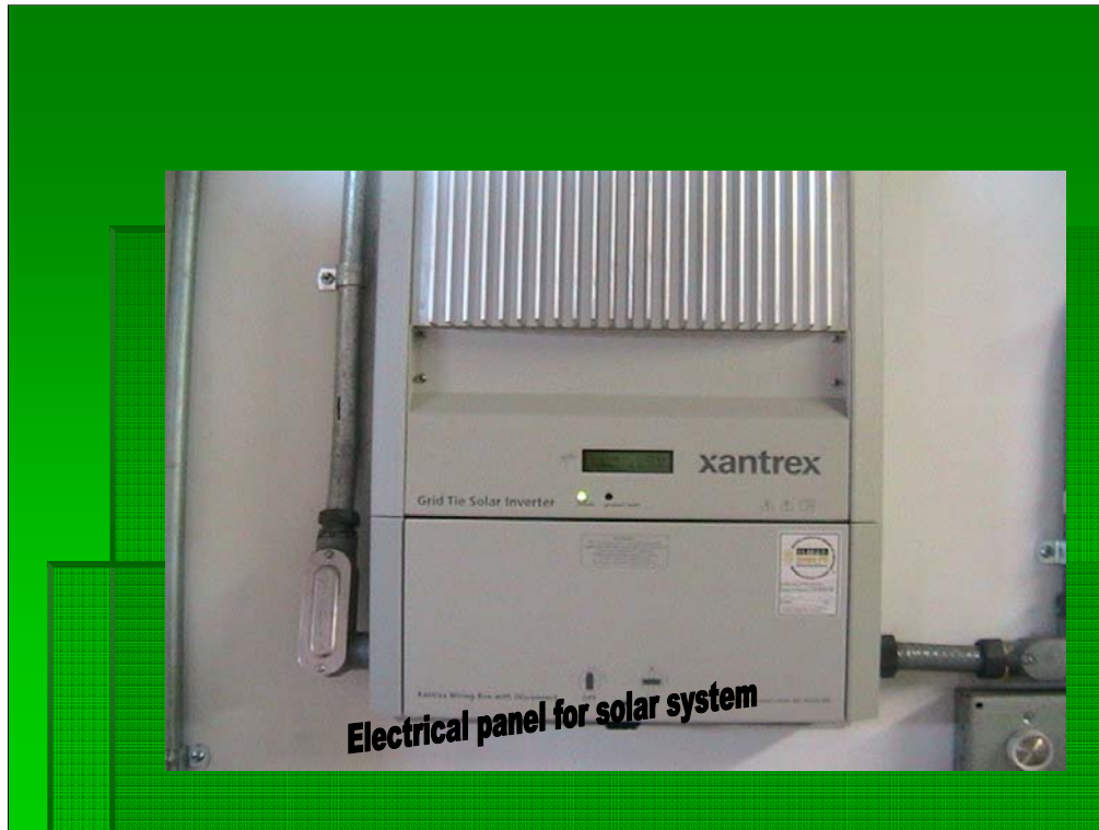
Electrical panel installed inside control room. Xantrax Grid Tie Solar Inverter owner's manual.
