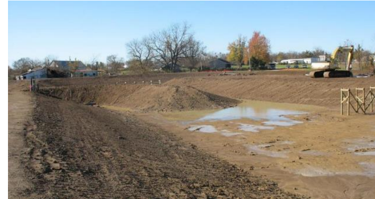
MRPTS oxidation cell under construction, fall 2008
