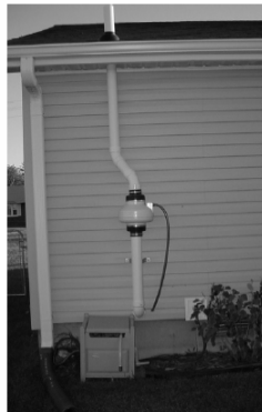
Figure 4-3. Active subslab depressurization system.
