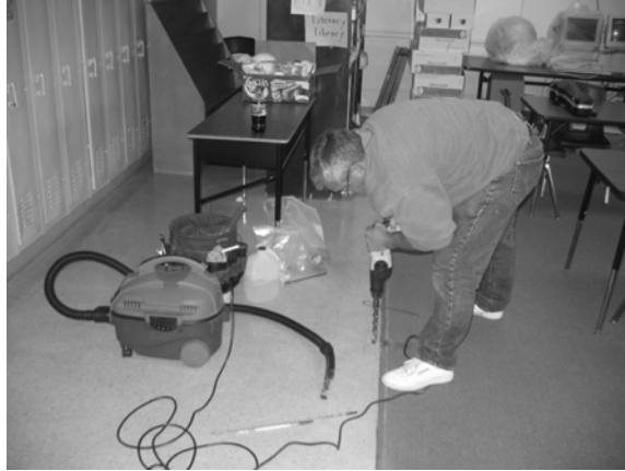
Drilling Through Slab
