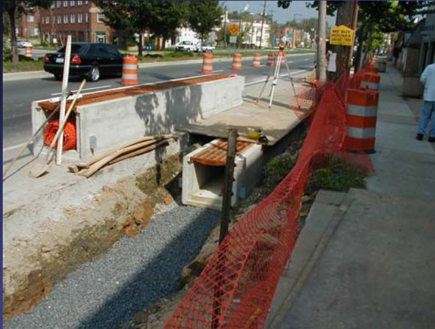
SHA Mt. Ranier Gutter Filters Integrated into Streetscape
