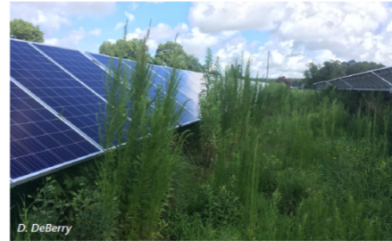
Figure 5-1: Solar facility in Virginia constructed on a prior agricultural field. This site did not use a Pollinator-Smart approach to vegetation management and, as a result, is dominated with aggressive weeds that are already overtopping the panels even before the first growing season is over.
