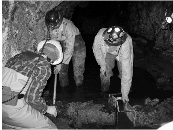
Setting a flume underground
