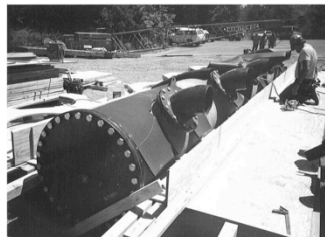
Multiport Diffuser Construction
