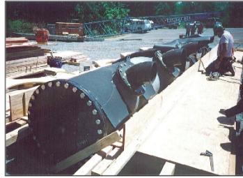
Multiport diffuser under construction
