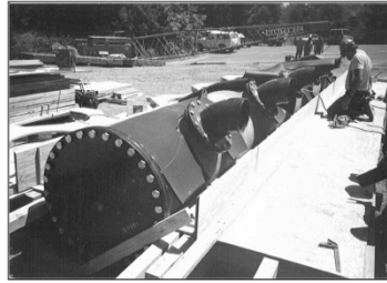
Multiport diffuser under construction
