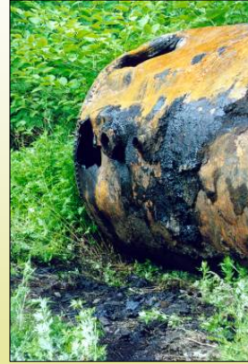
UST removal at Riverside Hills, Providence, Rhode Island
