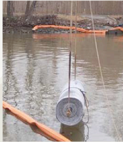
Placement on Subaqueous Sediment (courtesy of CETCO®)
