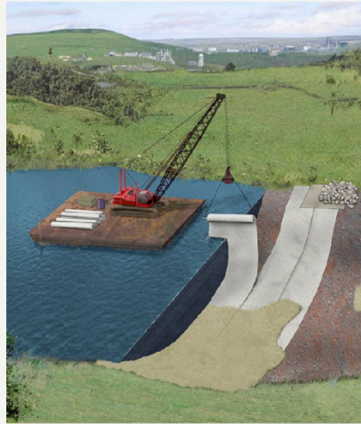
Placement on Subaqueous Sediment (courtesy of CETCO®)
