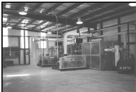
LFG Compression and Treatment Facility
