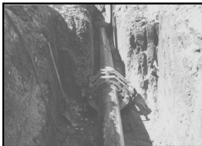
Pipeline to Rolls Royce 7200 ft. 12 inch HDPE
