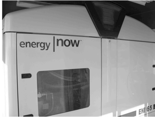
65 kW IPower Energy Systems Generator
