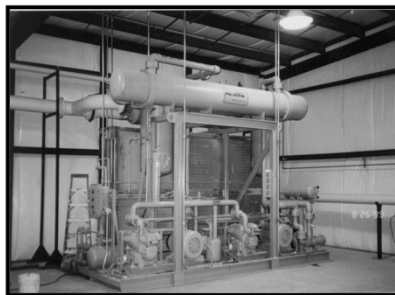
Pneumatech Refrigerated Gas Dryer
