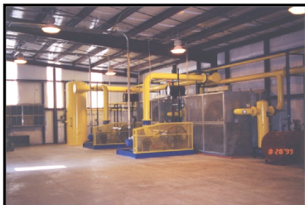
LFG Compression and Treatment Facility
