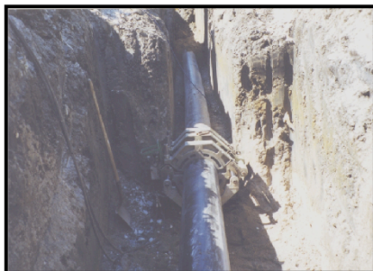
Pipeline to Rolls Royce 7200 ft. 12 inch HDPE
