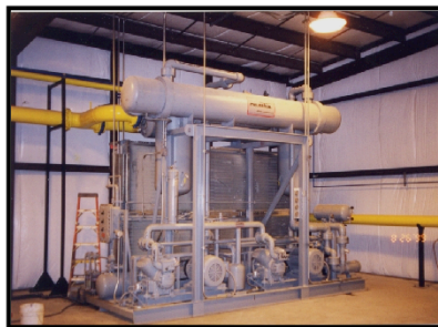
Pneumatech Refrigerated Gas Dryer
