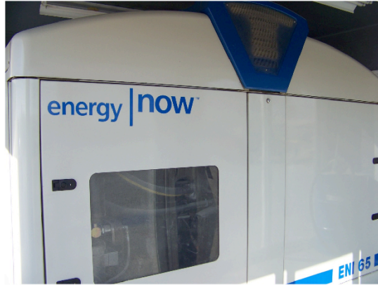
65 kW IPower Energy Systems Generator
