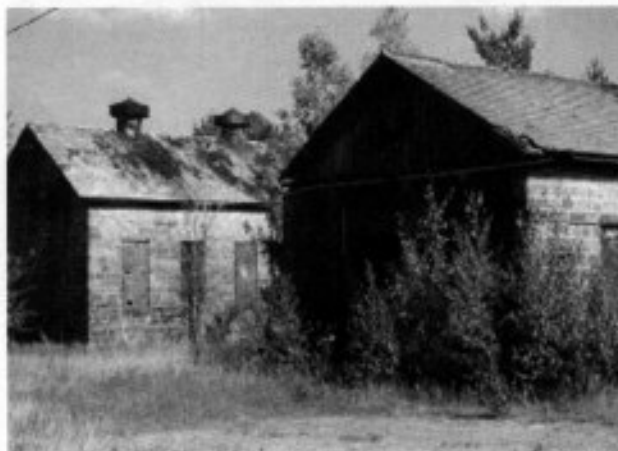
The machine shop and motor repair barn of the long-abandoned Reitz No. 4 mine is part of the nation's first coal-impacted watershed recognized as a brownfield.
