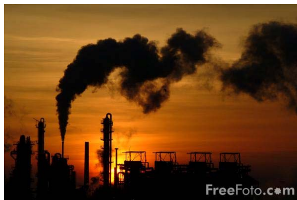
Industrial Process Control
