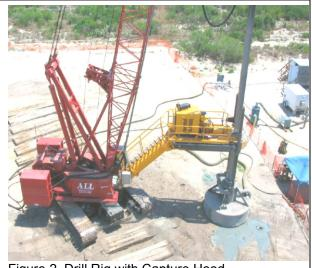
Figure 2. Drill Rig with Capture Hood
