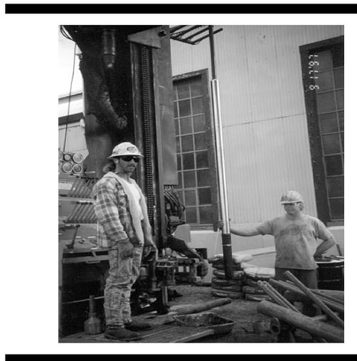
The Simulprobe™ provides continuous sampling of soil gas in the vadose zone. When the probe is pushed through the vadose zone, soil gas is extracted under the vacuum and measured continuously in an organic vapor analyzer located above ground surface. If desired, a syringe can be inserted and a sample of soil gas can be extracted and analyzed by gas chromatography (GC) at any time.
