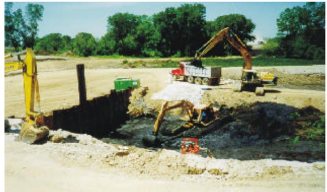
then excavating sediment using modified backhoes capable of maneuvering within the sediment bed of the Unnamed Tributary. Once the pre-defined removal depths were achieved, post-confirmation PCB sampling and (where determined necessary) additional excavation were performed prior to backfilling.
