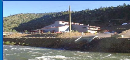
Argo Tunnel After Remediation
