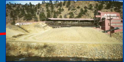
Runon/Runoff Control at Waste Rock Piles
