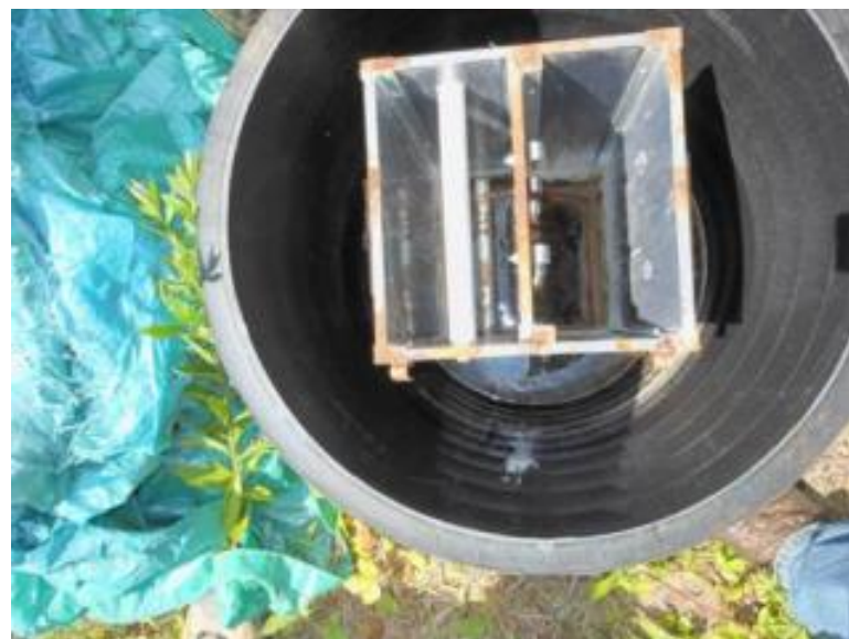
Adjustable Elevation Head Weir for BCR Effluent
