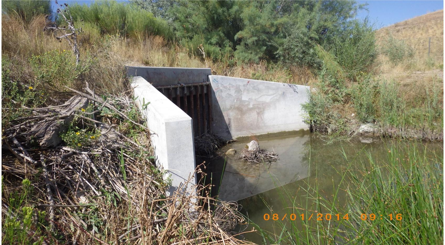
2009-EPA installed two design build box culverts to increase holding capacity of river
