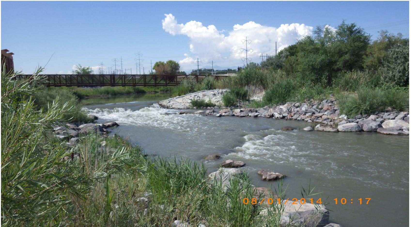
2014-Grouted boulder structure repaired with two added cross-veins to aid in navigability
