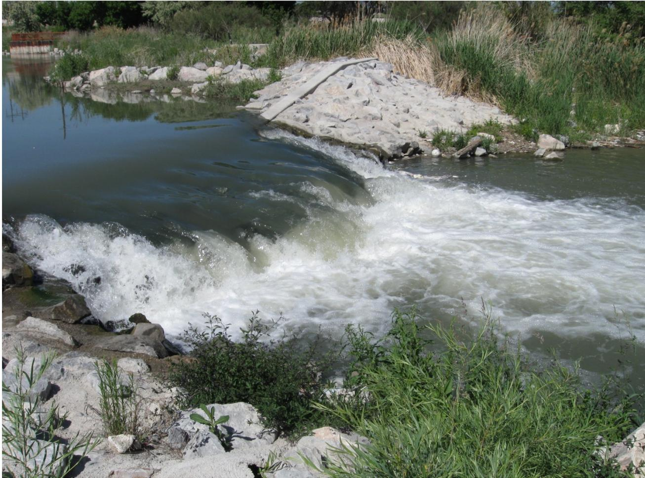
2010 and 2011- High Flows cause damage to the grouted boulder structure
