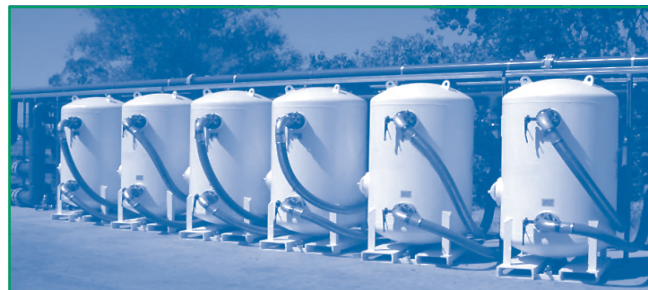
Figure 3. The Rancho Cordova ion exchange system employs a "6 by 6" matrix of treatment vessels collectively containing 720 ft 3 of styrene-based resin.
