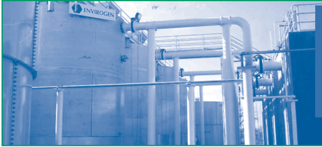
Figure 2. The $5 million FBR at Aerojet's Rancho Cordova facility operates 24 hr/day, 7 days/week to remove perchlorate from ground water.
