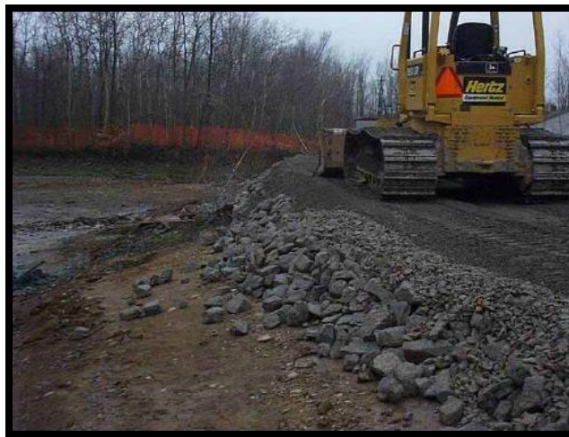
Figure 5: Roadway at Barker Chemical Site
