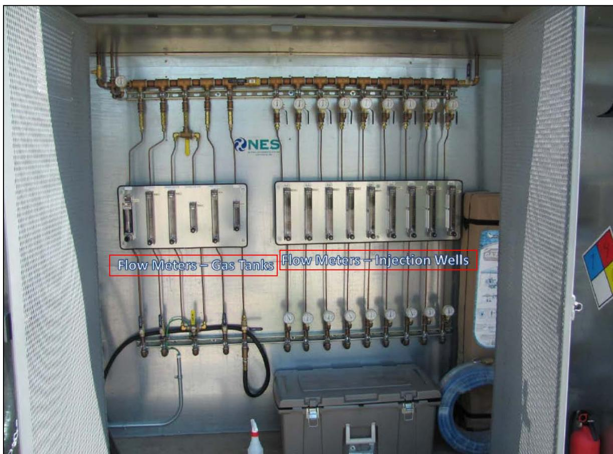
**Figure 23:** Gas mixing (left side) and injection (right side) skid for the H<sub>2</sub>T system
