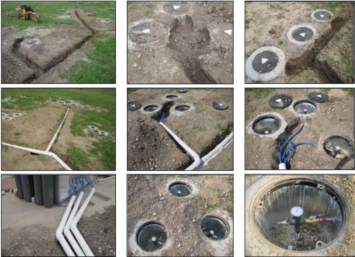
**Figure 26:** Trenching, piping and wellhead installation for injection wells
