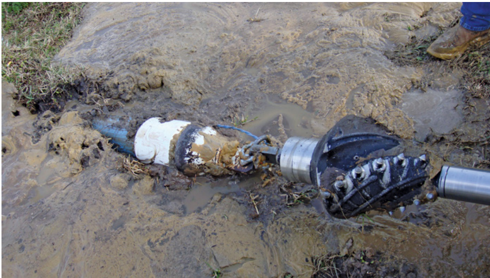
Exhibit A-19. Back Reamer (Right) Attached To Well Casing (Left) After Pullback
