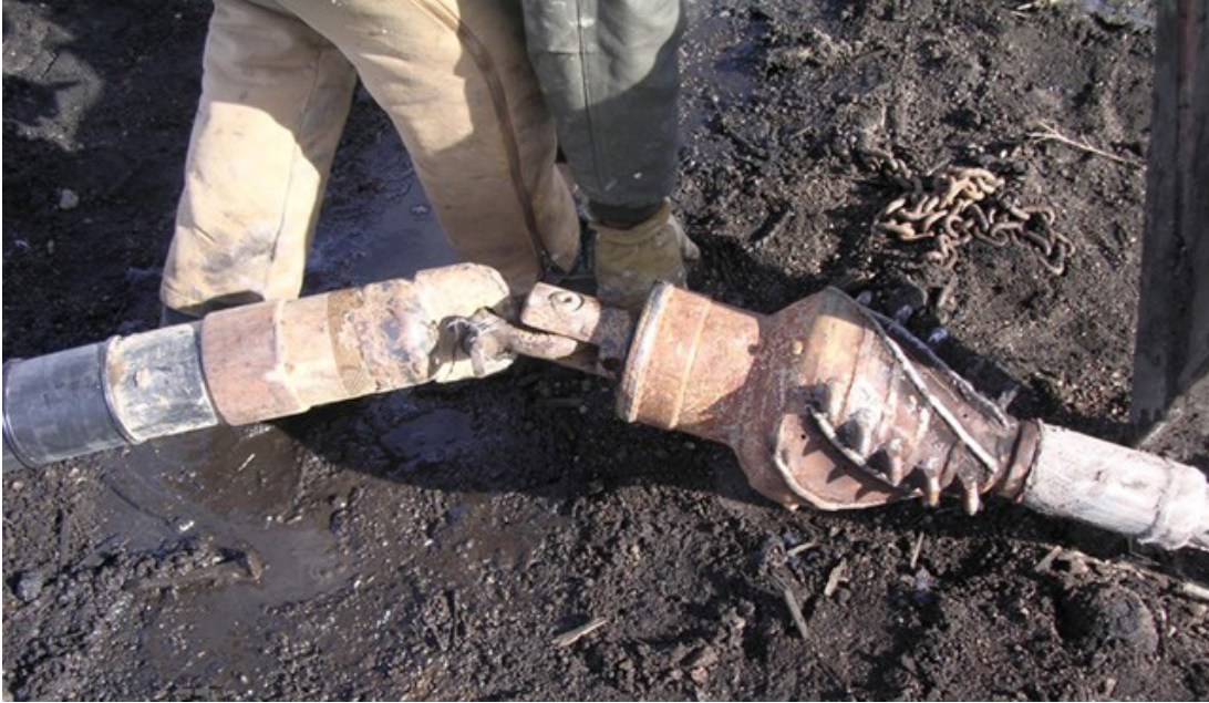
Exhibit A-18. Back Reamer (Right) Attached To Well Casing (Left) Prior To Pullback
