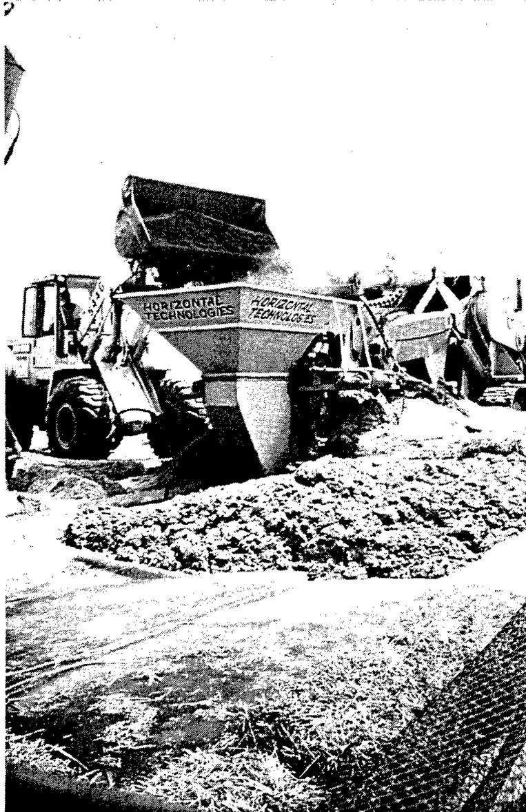
**Figure E-6. Continuous Trencher Simultaneously Excavating a Trench and Refilling it from Behind with Granular Iron, Elizabeth City, NC (ETI, 1997)**
