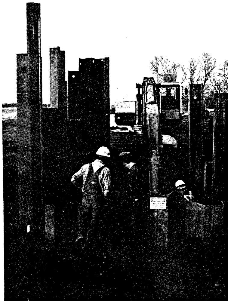
**Figure E-2. Initial Excavation of a Gate in the Center of the Slurry Funnel Wall, DOE Kansas City Plant (ETI, 1997)**
