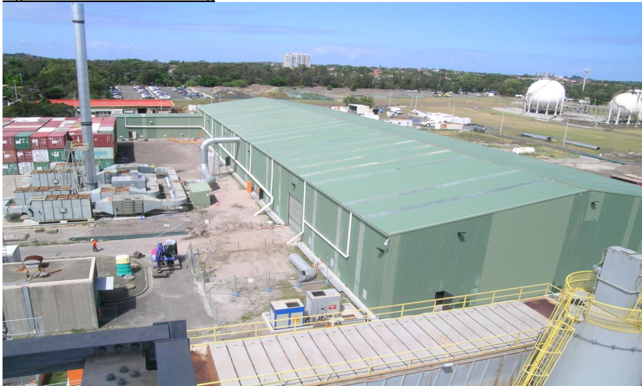
Figure 1: The Feed Soil Building
