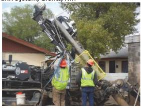
Figure 6. Sheet pile Electrode Installation
