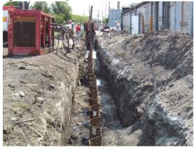
Figure 7. Horizontal Electrode Installation
